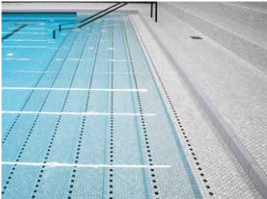
School swimming pool Vogelsang of the primary school, Basel, Switzerland Architect: MET Architekten GmbH SIA, Basel, Switzerland Series: Pool edge system Wiesbaden, Swimming pool special programme, Chroma Pool, Loop Photo: Daniel Zehnder
