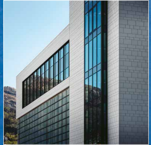
Hytect cleans the air of pollutants such as NO x Fabrikkgatan, Bergen, Norway / Architect: Ramboll Norge AS Div / Photo: Morten Wanvik
