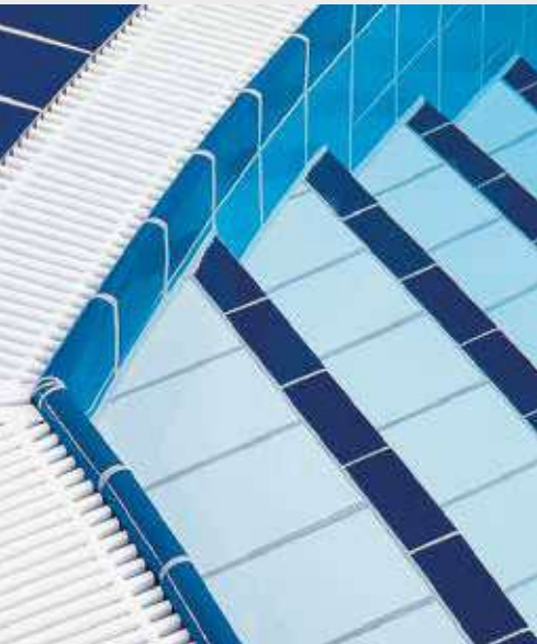
Ins Wasser führende Treppe mit Radialleisten-Vorderkante Stairs leading into the water with front edge executed by means of radial corner pieces
